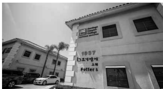
OEC Provisional Education Facility (CHAP) Tel: 714-628-5900
